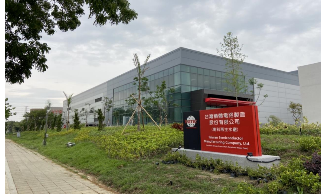
TSMC Southern Taiwan Science Park Reclaimed Water Plant
