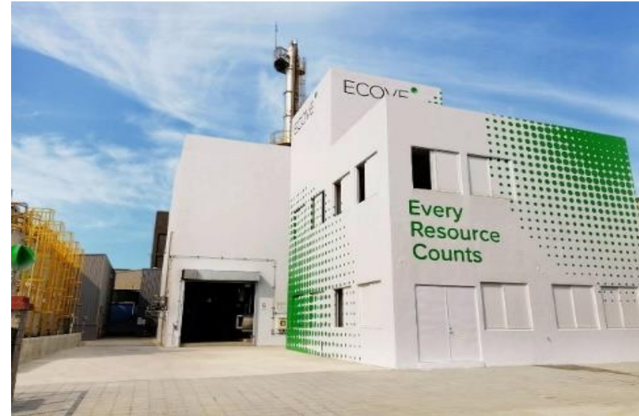
ECOVE SRC Waste Isopropanol Recycling Plant
