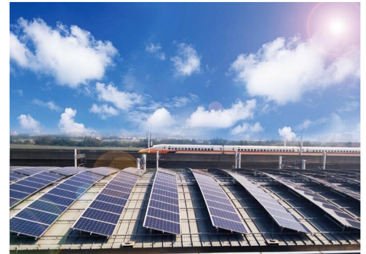
THSR Yanchao Solar Power Project
