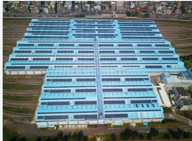
Taipei Changxing Solar Power Plant
