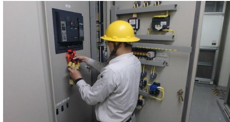
MCC equipment maintenance and power outage operation
