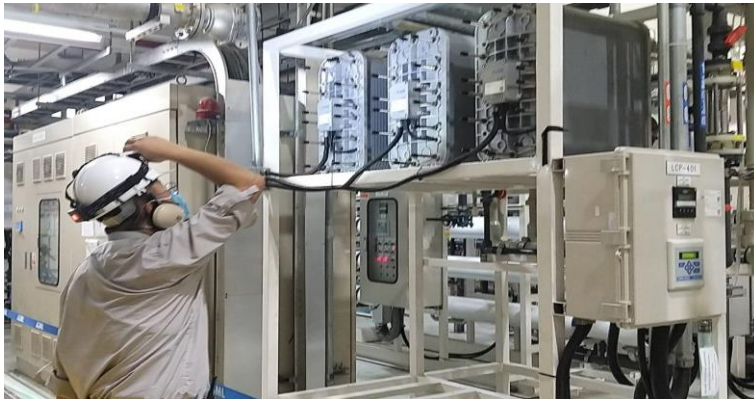
Inspection of Chiller Room
